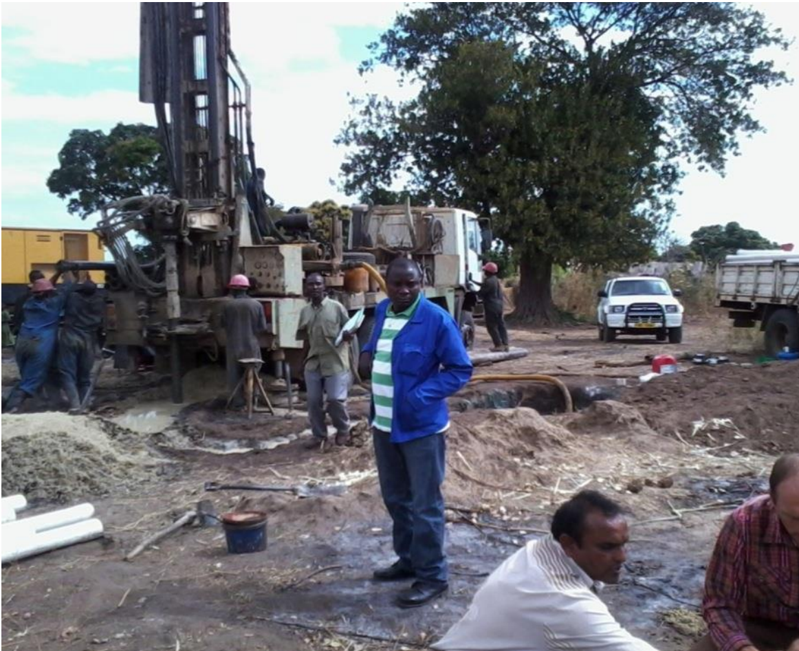
Photo 14: Borehole drilling works in a village in TA Sitola, Machinga
