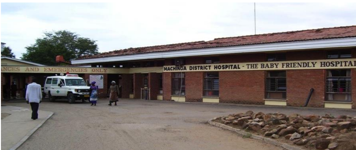
Photo 11: Machinga District Hospital, The Baby Friendly Hospital.
