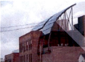
Sarunac Building: Consider how a project can take advantage of green technology effective in Spokane's climate.
