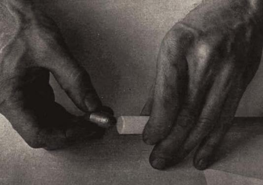
Heavy .57 caliber bullet is inserted point first into rolled paper tube containing powder charge. Tube is then crimped at ends.
