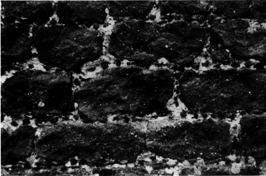
Fig. 4 Carstone wall galleted with carstone. Kingsley, Hants, Old Church (SU 788 382)
