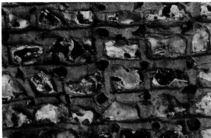
Fig. 7 Flint wall galleted with flints laid flat. Churchyard wall at West Dean, West Sussex (SU 861 126)
