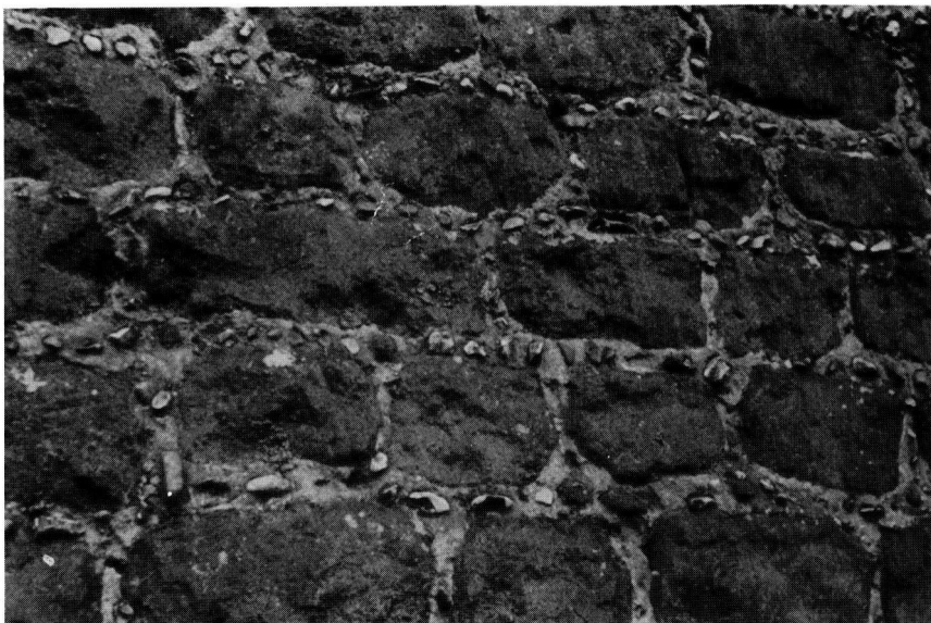
Fig. 10 Carstone wall galleted with pebbles. Barn at Heacham, Norfolk (TF 675 373)
