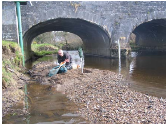
Plate 6.10. Bonet River, New Bridge, Co. Cavan (LE2).
