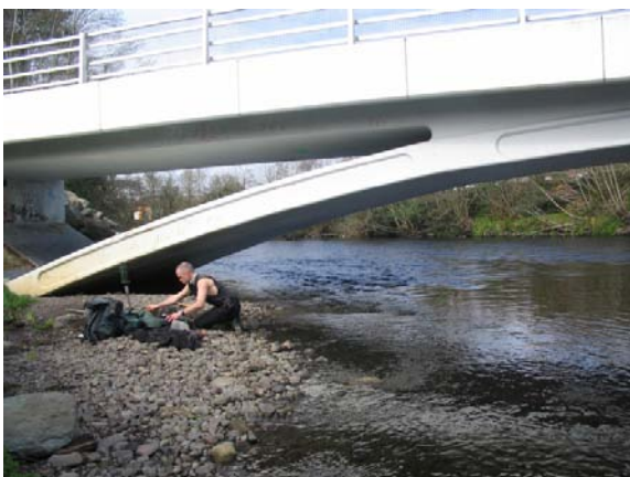
Plate 6.11. River Flesk, Ballyspillane bridge, Co. Kerry (LE2).
