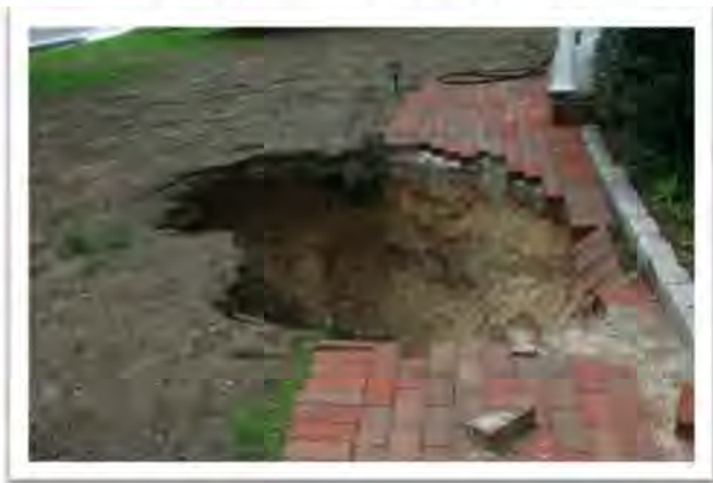
Figure 4. Collapsed cesspool.
