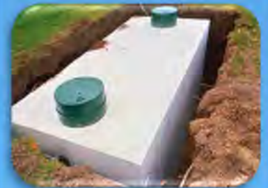
Figure 2. Installed septic tank.
