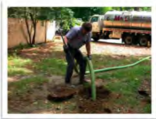
Figure 4. Pumping of septic tank.
