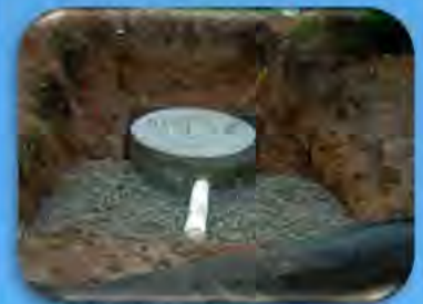
Figure 2. Uncovered cesspool.
