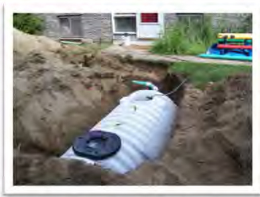
Figure 3. Newly installed septic tank.
