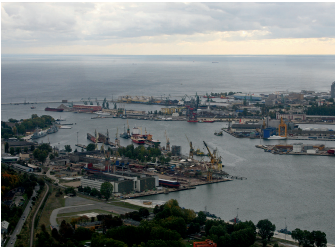
Estuaries have been severely affected by construction activities in the Baltic Sea region, historically harbours were often established in these areas. Photo: Maritime Office Gdynia.
