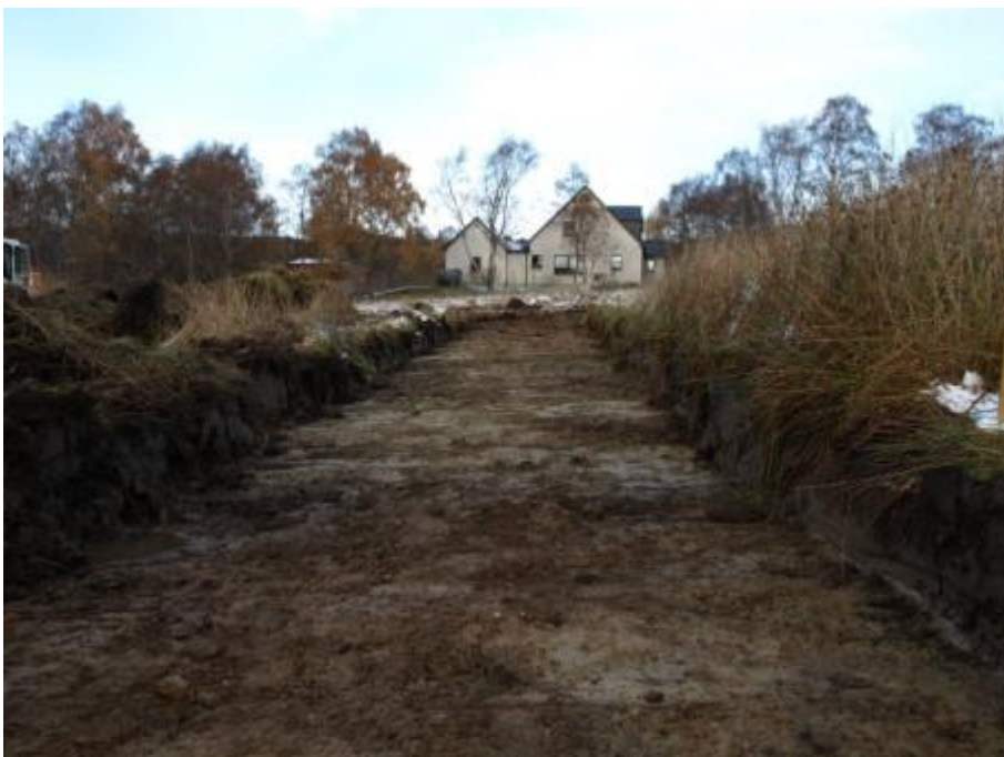
Figure 8 Area 4 stripped. Photograph 21.
