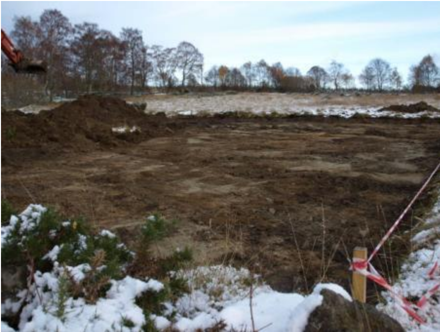
Figure 7 Area 3 stripped. Photograph 25.
