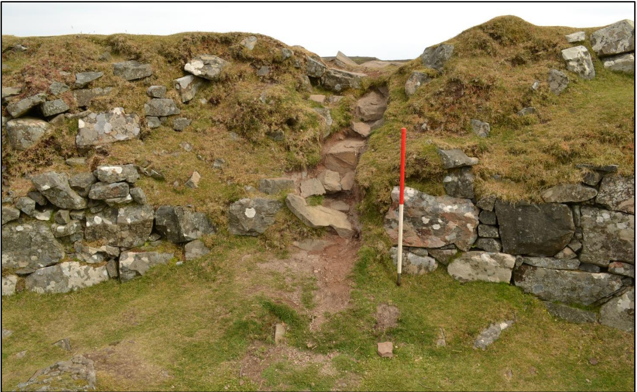
Plate 3: Erosion on inner broch wall, Site 36, facing NE.
