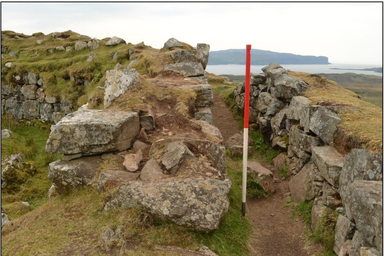
Plate 4: Erosion on the broch wall head, Site 36, facing SSE.
