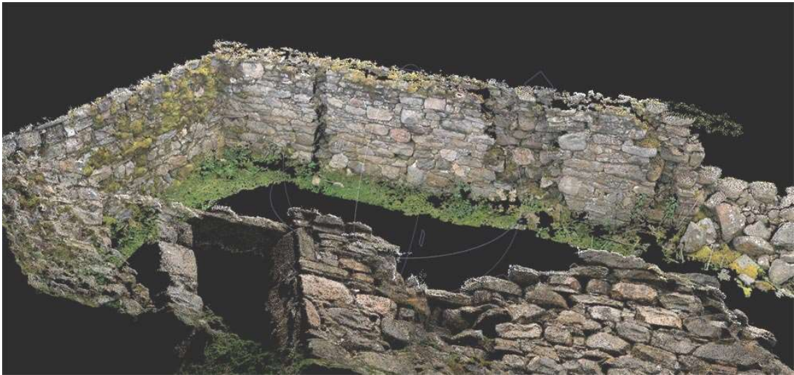
3D model of the internal faces of the 1840s building showing cruck slots
