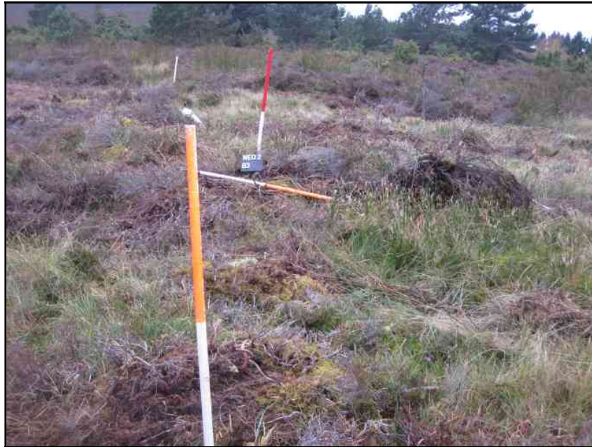
Building footings, B3
