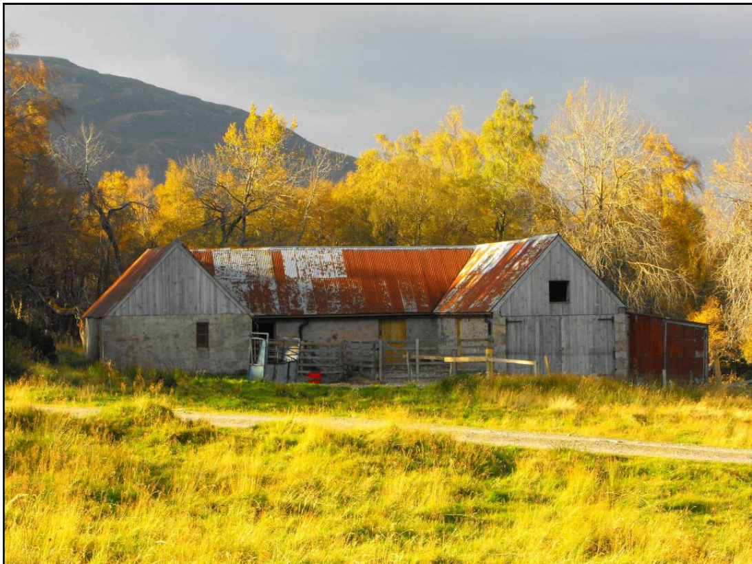
The late 19 th century barn at Chapeltown (photo courtesy of Richard King). Barn of has corrugated iron roof like the 1880s building and part wooden gabled walls like the latter's NW gable.
