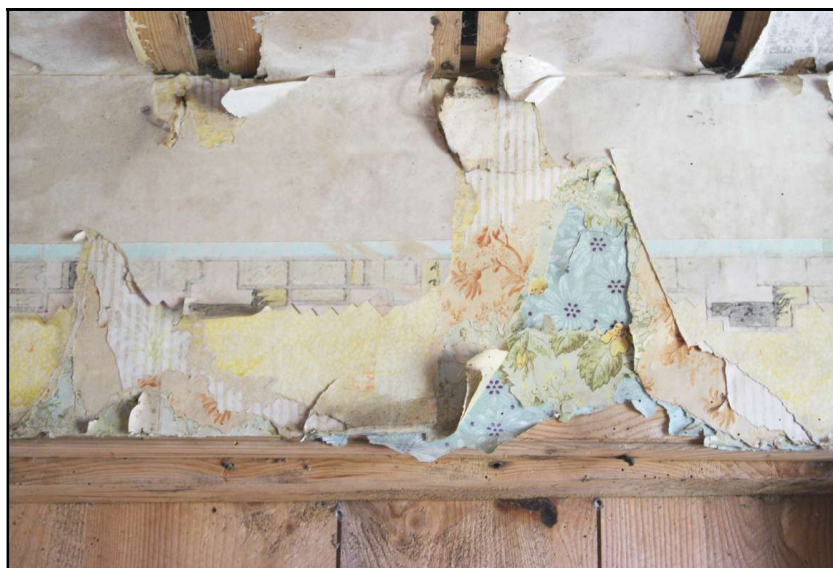
Photo of the 6 different layers of wall paper in the NE room
