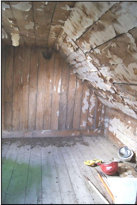
The NE room, 1 st floor
