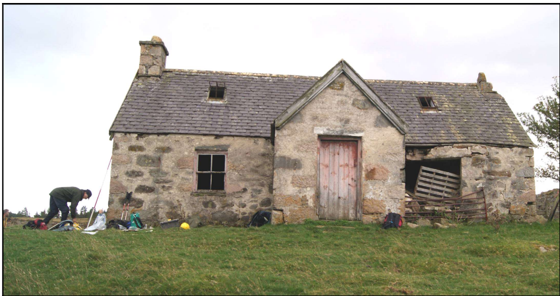
General shot of the front elevation
