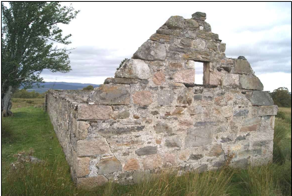
The Gable wall of the 1880s building
