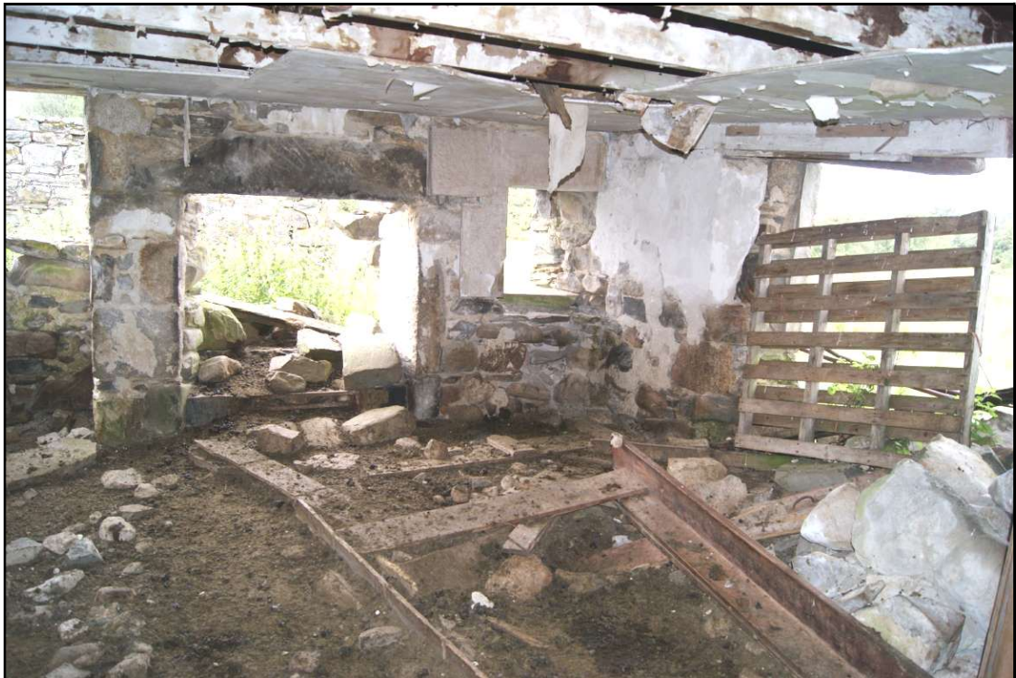
Shot looking at the SW room
