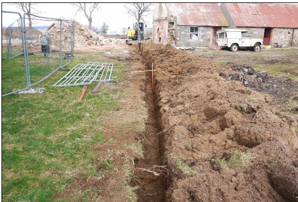
Figure 10 – The electricity supply trench during excavation. Facing N. Scales 1m
