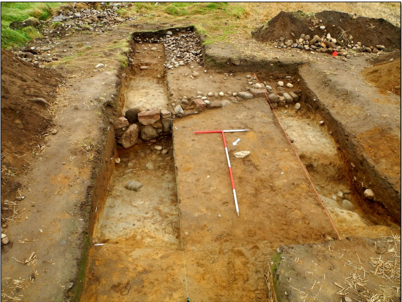
Plate 33 – View SE over Trench 2a extension showing revetment wall F2.04 and ditch cut [2.16], with field clearance stone visible within uncultivated area of ground at far end of trench
