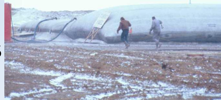
Fuel storage bladders
