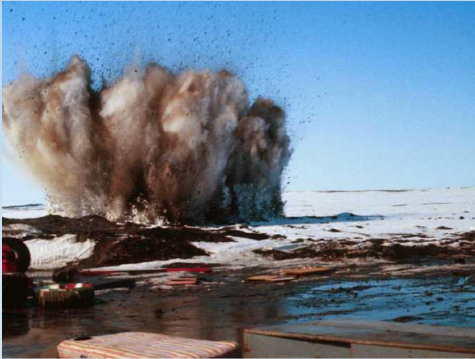
Digging a Pit in Permafrost
