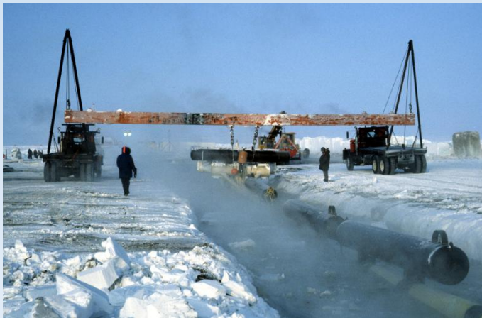
Laying pipe through ice trench
