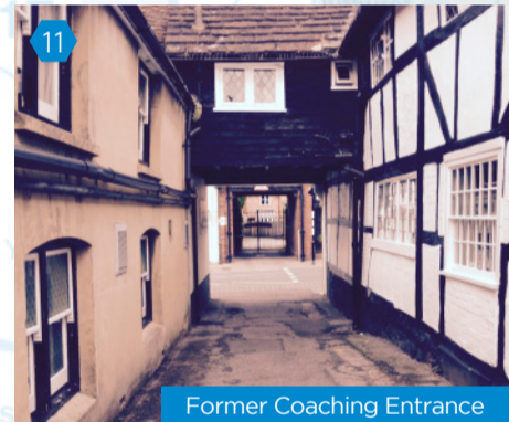
Former Coaching Entrance
