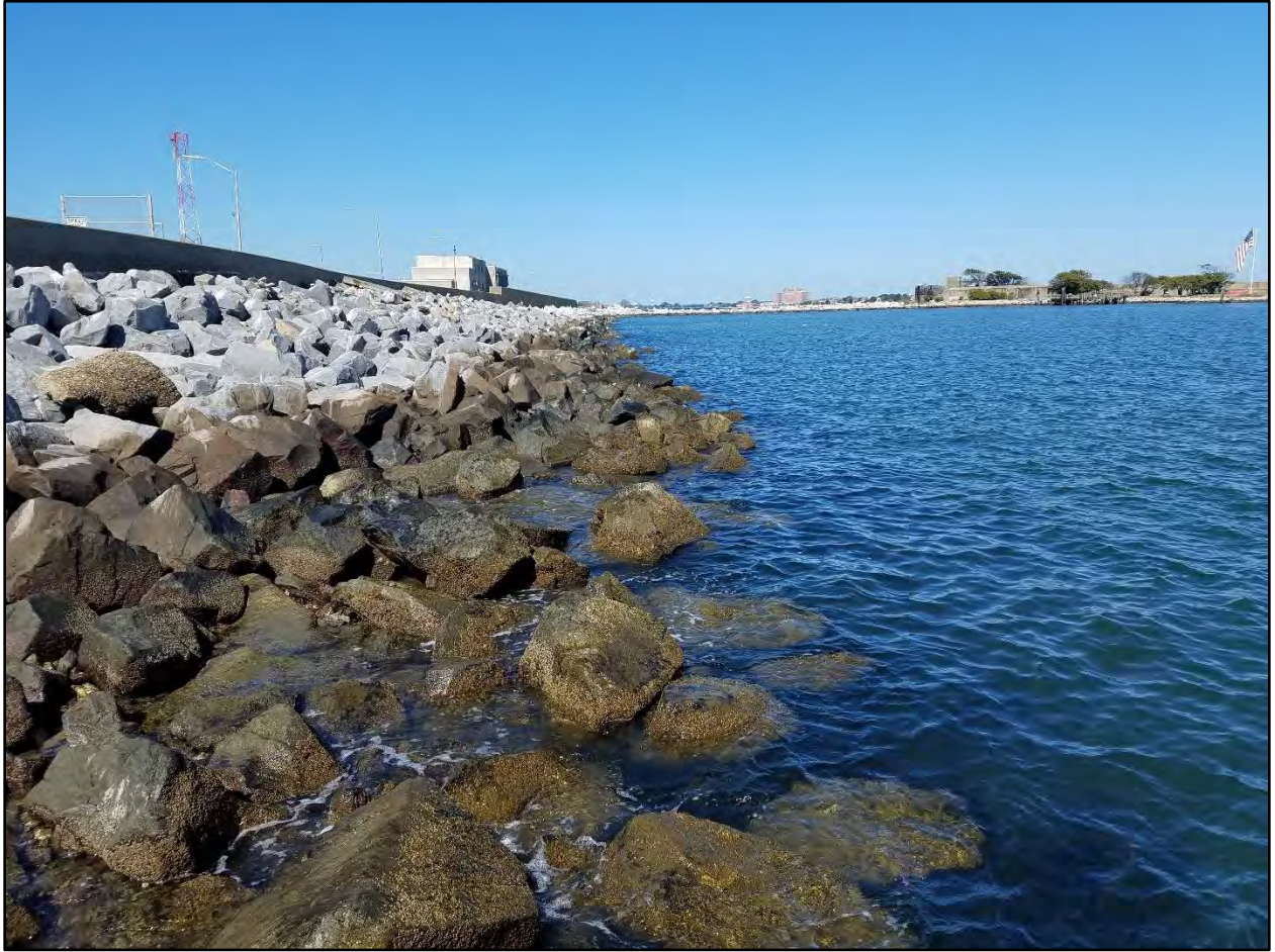
Figure E-1. Rocky shoreline of the southern portal island of the HRBT. Intertidal samples were collected among the rocks during the portal island benthic survey
