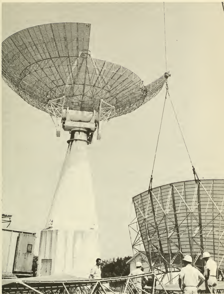
The 84-foot steerable dish shown here being taken apart at Huntsville, Alabama, is now being installed at the Agassiz Station in Harvard, Mass., where it will replace the 60-foot one formerly at Agassiz and will sit on the same pedestal and be operated by the same machinery.
