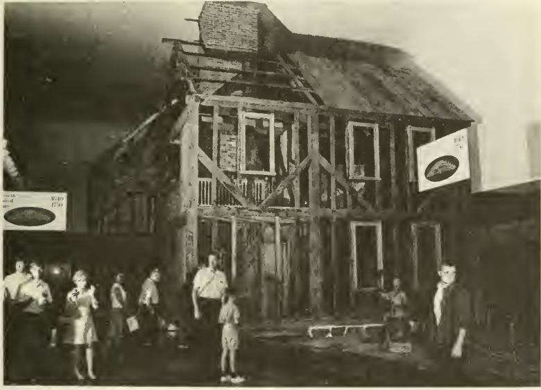
The two halls opened in the growth of the United States series cover the period 1640-1851. Construction methods used in 1690 and 1750 are illustrated by this house from Ipswich, Massachusetts. Below: Two-man pit saw used to rip out planks.
