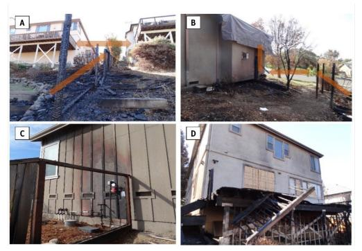
Figure 9: Examples of structural fuel connectivity and the role in damaging the main building in a parcel during the Glass Fire. A combustible fence (A and B) supported flaming ignition, moving from downhill all the way to the main building, and caused severe damage (C and D). A and B are annotated with arrows representing the estimated direction of fire spread.
