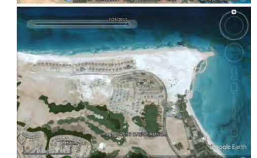
Marassi resort development in a dune / sabkha system facing a highly dynamical barred beach.
