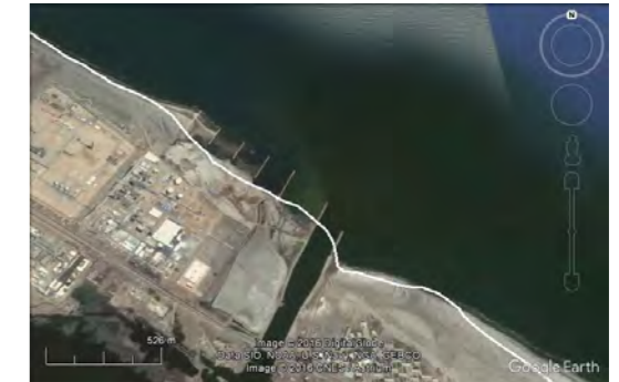
El Gamail strait: siltation issues and construction of new sea groins. Top: 2009, bottom: 2016.
