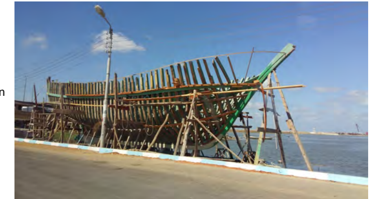
Ship construction works, Burullus fishing port.
