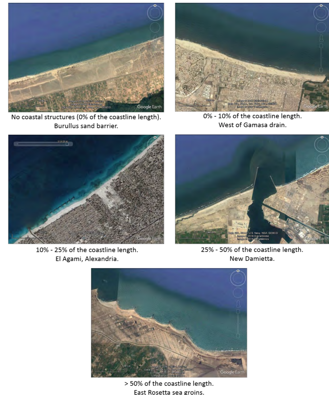
Percentage of coastal stretch affected by coastal structures: the Human Disturbance Indicator (HDI).
