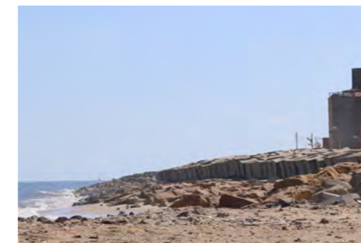
Coastal protection works on the coastal front in the Delta apex.
