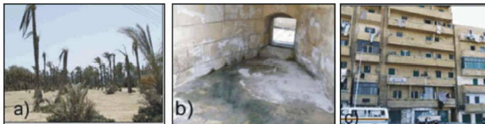
Fig. 17: The effect of rise of Mediterranean Sea and groundwater levels on study area; a) death of palm trees in Rashid; b) chemical weathering on the floor of Rashid Bay Citadel; C) distraction and inclination of building.
