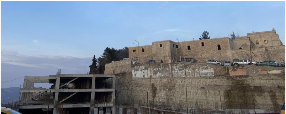
Figure 4. A Scene From Shopping Mall Construction and the Texture of Old Mardin (Eda Koçak's Personal Archive, 2022)
