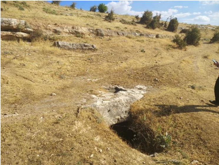
Figure 5. Image of the Entrance Door of the Water House (Original, 2019)
