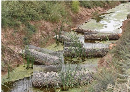
Figure 4. Screened Artificial Wetland Pilot Project to Improve the Quality of Water Returning from Irrigation" by the General Directorate of Water Management of the Ministry of Agriculture and Forestry
