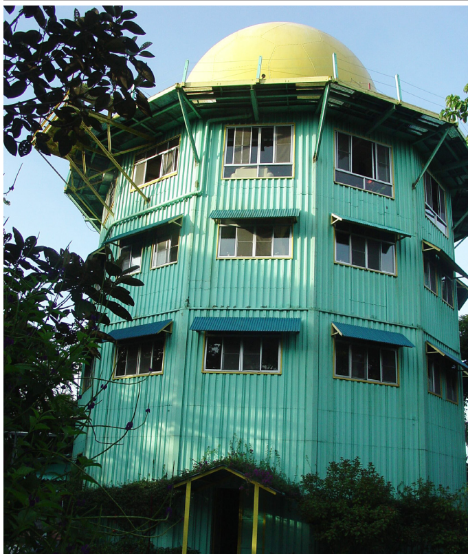
Canopy Tower with radar dome on top.
