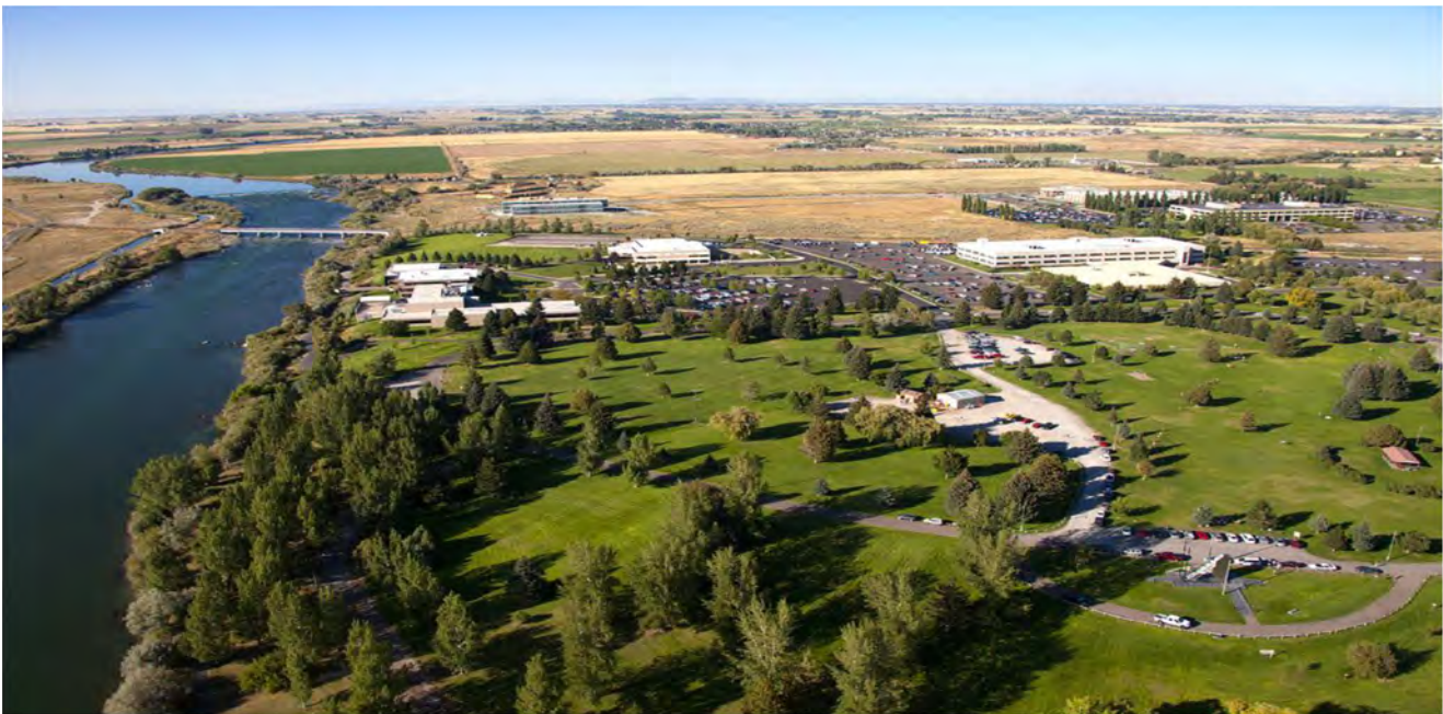
Figure 3-1. BEA's Idaho Falls Campus.
