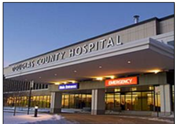
Douglas County Hospital – Alexandria, MN
