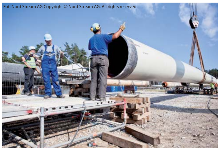
Fot. Nord Stream AG Copyright © Nord Stream AG. All rights reserved
