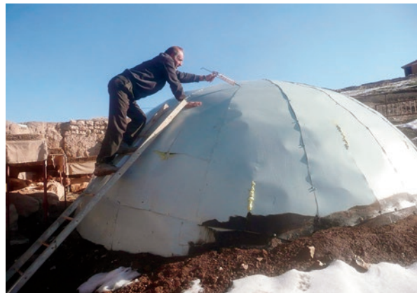
Figure 16. The new metal cover for the abi in the fall of 2013.
