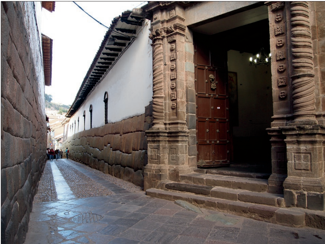
Figure 4. The entrance to a colonial building built into a former Inca ritual platform.
