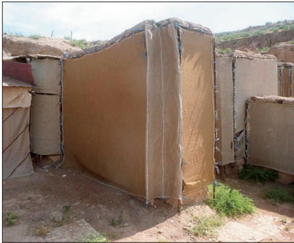
Figure 11. An “arte povera” approach to wall conservation: individual panels replacement.
