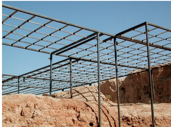
Figure 8. Detail of trellis, showing modularity of system.
