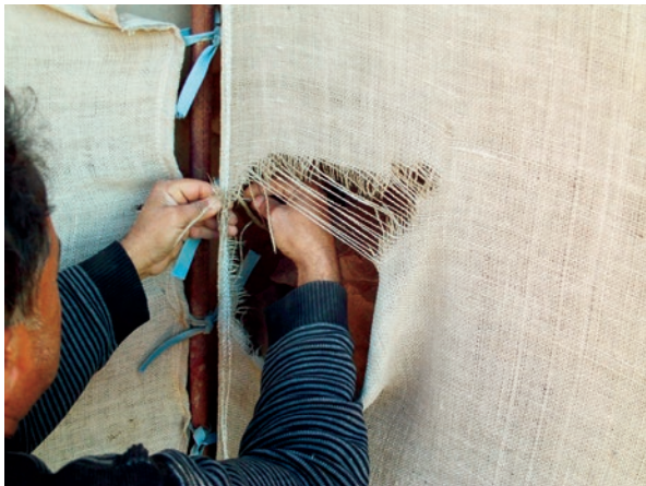
Figure 12. Patching of holes in panels.
