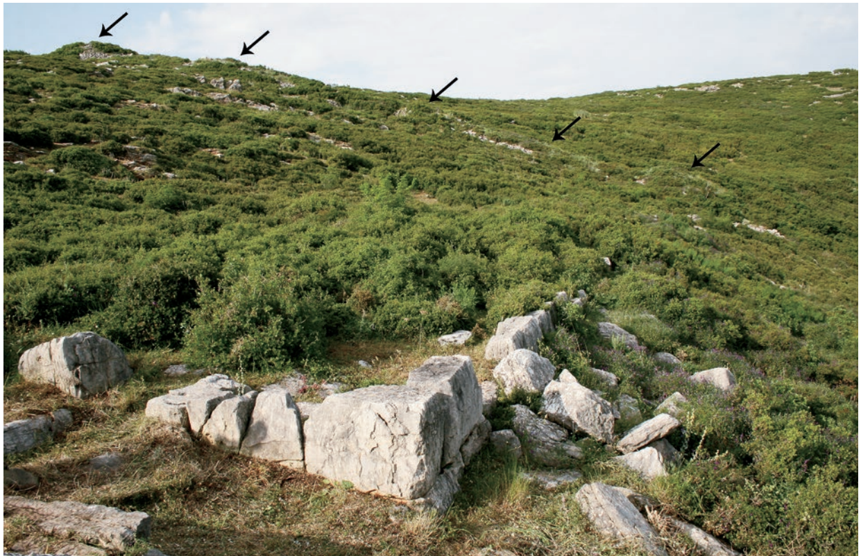
Figure 4. Postern V in the foreground with the remains of the diateichisma visible in the background. Note the poor level of preservation and heavy overgrowth.
