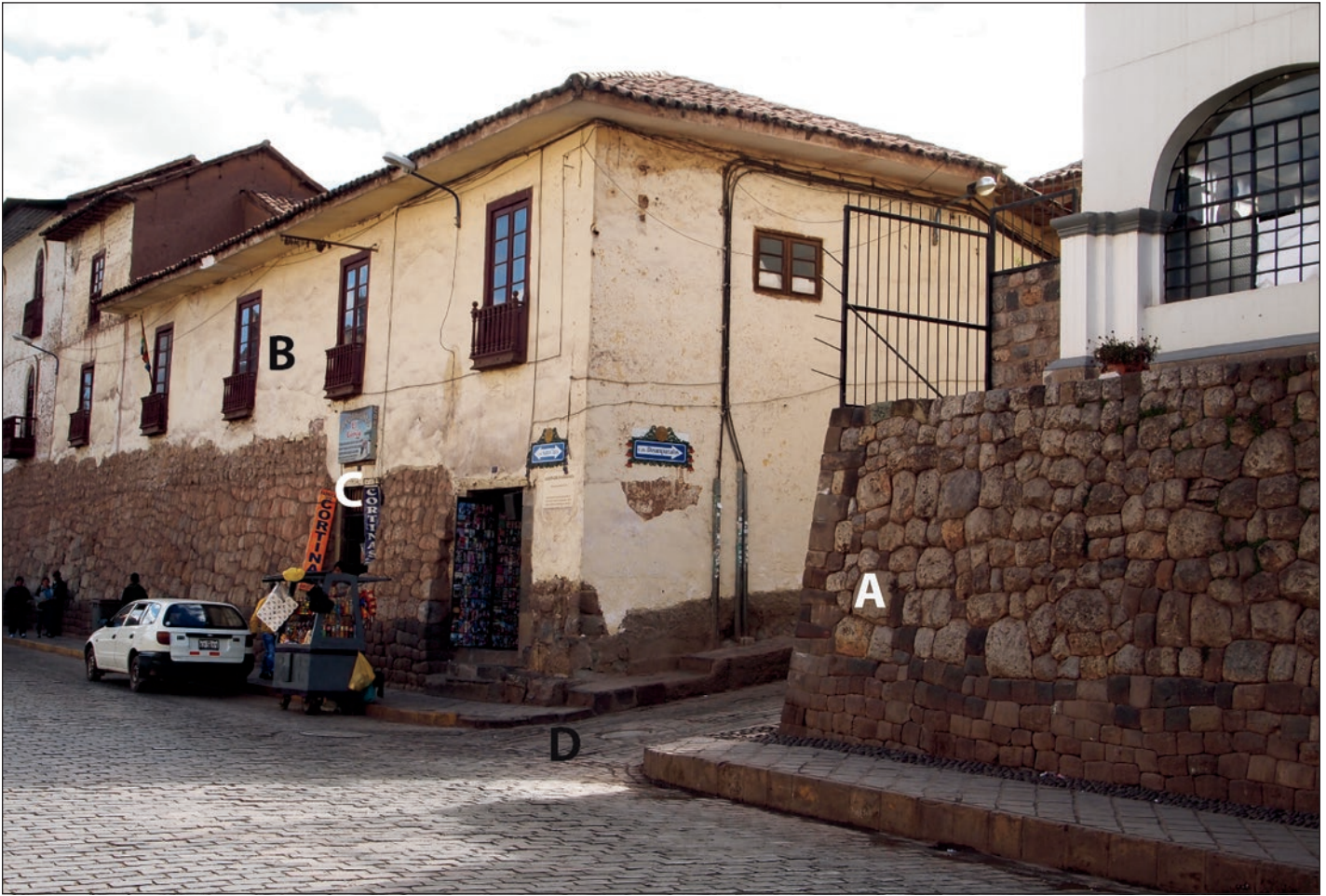
Figure 5. View of a monumental terrace revetment (A) that runs along the present market of San Pedro; (B) modern building on the approximate surface of the terrace; (C) modern store formed by vacating the fill behind the terrace; (D) original location of an Inca street.
