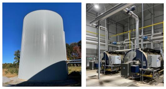
Figure 7. (Left) Hot water holding tank, and (right) boilers for heating the facility.
