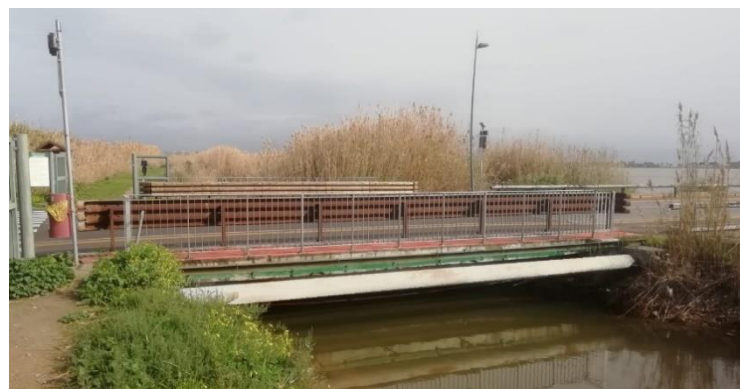
Figure 2. Bridge on Perdalonga canal Quartu Sant'Elena (Sardinia, Italy).
