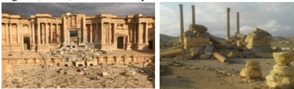
Figure (28-29)the damaged Stage, Figure ( )the damaged Tetrapylon
