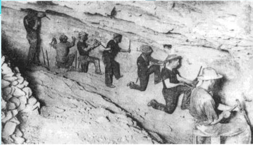
Single jackers working in a stope in the Goodenough Mine, circa 1880. Macia-Devere Collection
