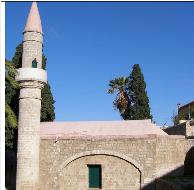
Pl.( 12): Mosque and minaret of AljalshnyTakiyya known as Barasani Mesgdi
