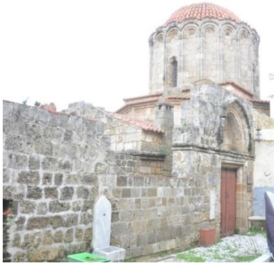
Pl. (7): The western facade of Agios Georgios Monastery (Chourmali Mosque).
