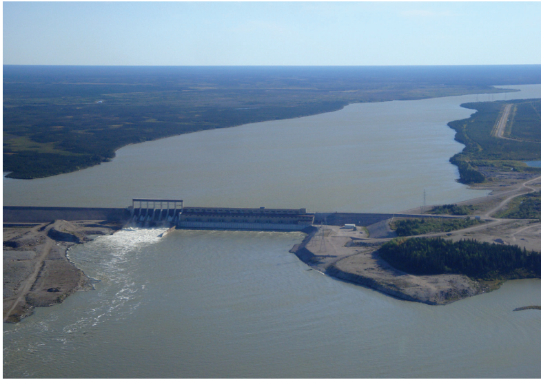
PHOTO 7-21 Aerial view of the Limestone Forebay.
