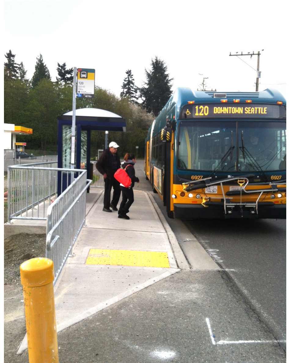
Guardrail at a Raised Landing Pad
