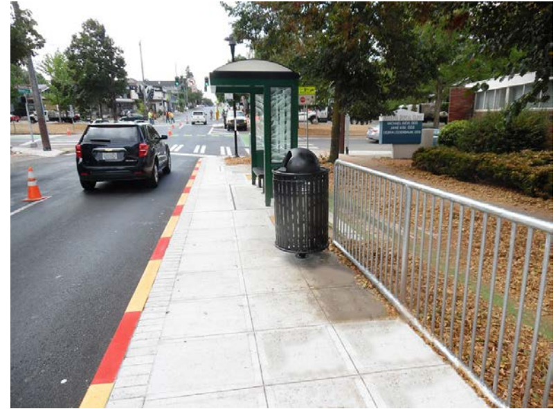
Bus Zone Curb Painting
