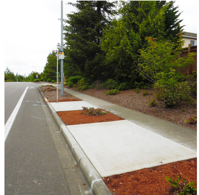
Landscaping between Landing Pads
