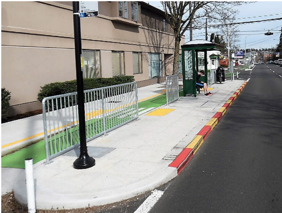
Guardrail at Transit Island
