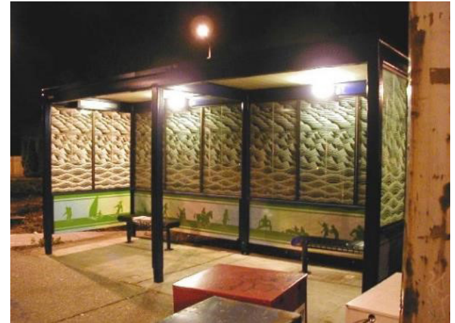
Standard Shelter with Lighting
