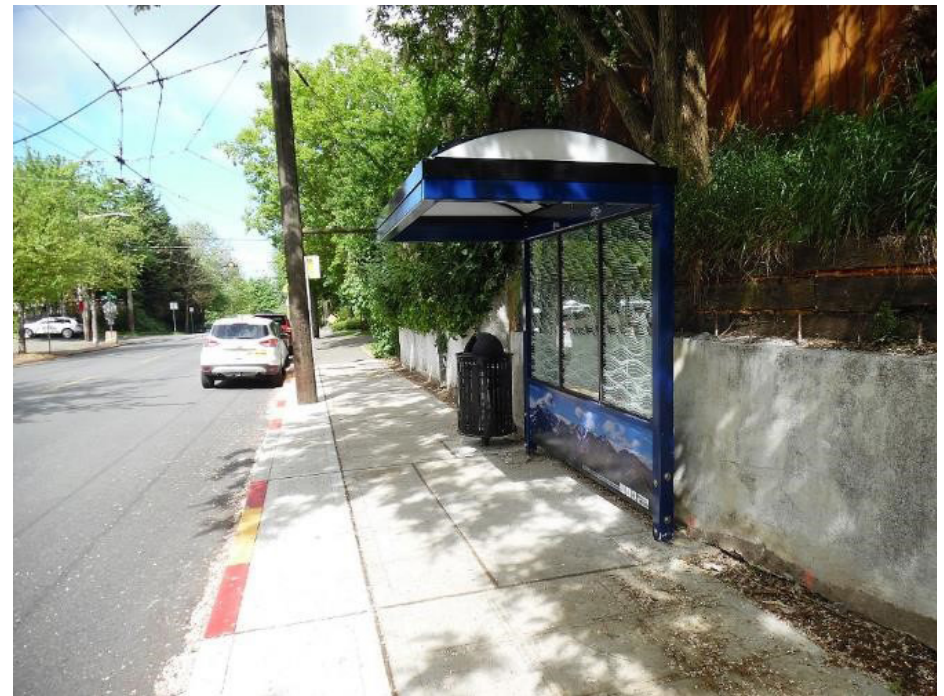
Shelter without Side Panels
