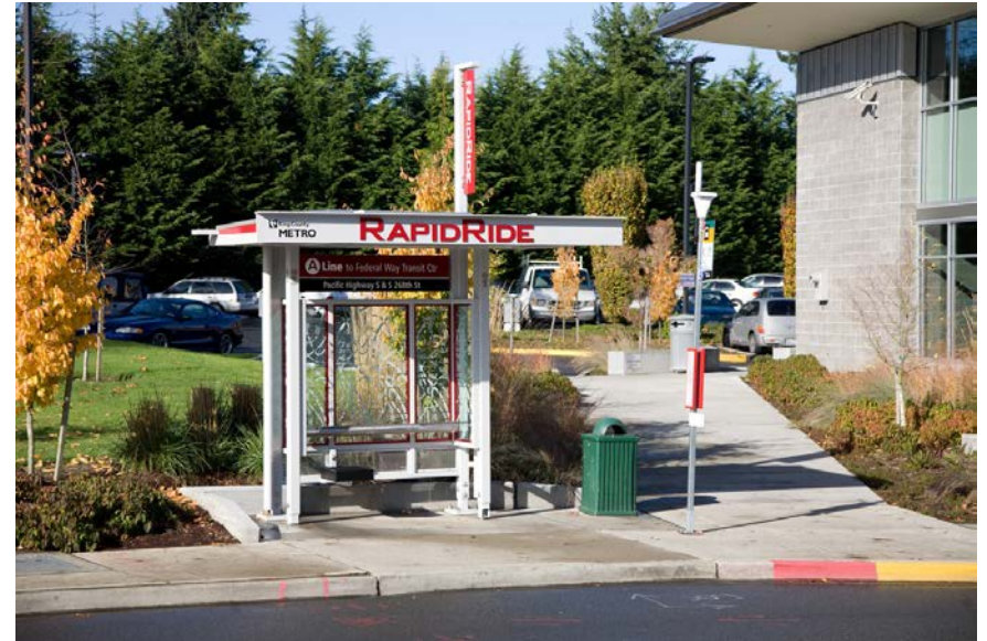
RapidRide Shelter at an Enhanced Stop
