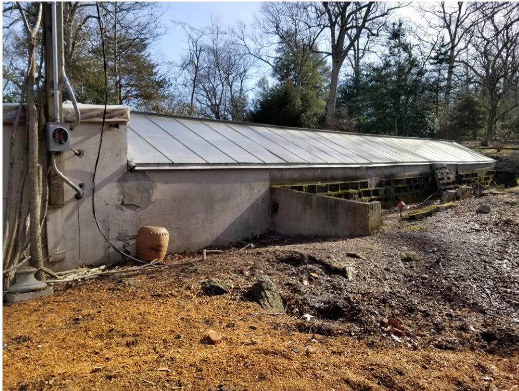
Upper Greenhouse Before Demolition
