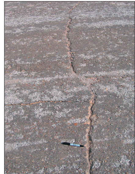
3a. Sample Cracking in Microcracked Pavement (top)
