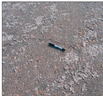
3a. Sample Cracking in Microcracked Pavement (top)
