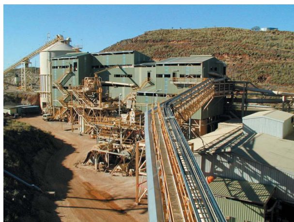
Figure 21. Ore-processing operations at the Wodgina mine. Conveyor feeds minus 12 mm tantalum ore to the upgraded primary-concentration plant
