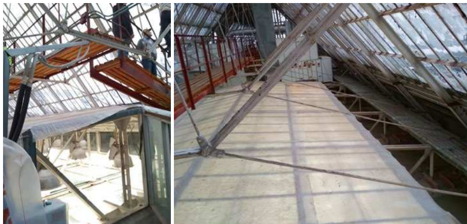
Fig. 10. Inner space and exterior of the sub-lantern
