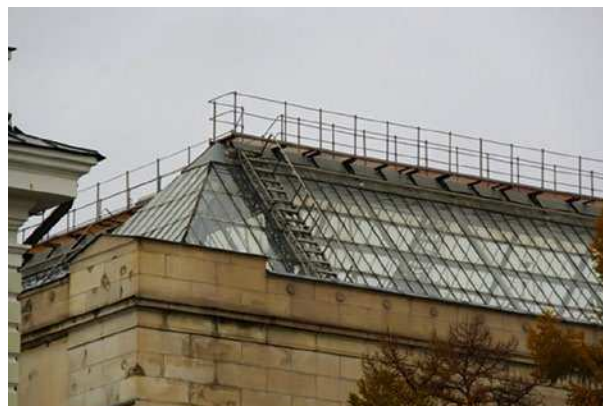
Fig. 6. Exterior of the transparent structure in 2018
