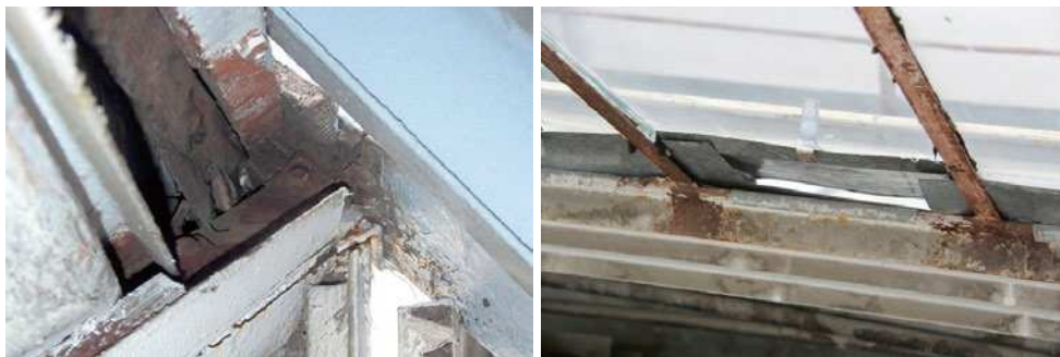
Fig. 7. Elements of the lantern light structure in 2018
