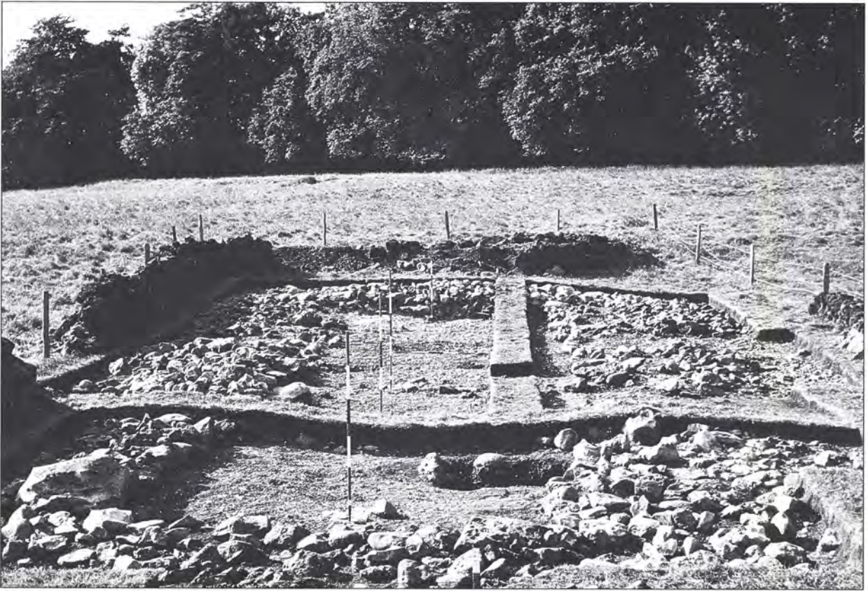
Plate XLIV Raddun: Building 1 from the south, showing how a platform has been made on the southerly slope to take the two-phase house, the newer end of which is nearer the camera
