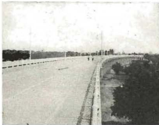
New Tuolumne River Bridge
