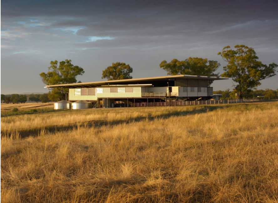
Fig. 4.8 Deepwater woolshed in New South Wales, Australia
