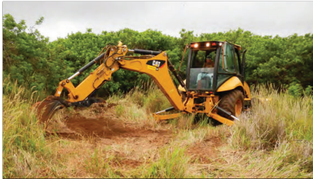
Figure 79: Excavation of Test Pit 22, looking southeast.
