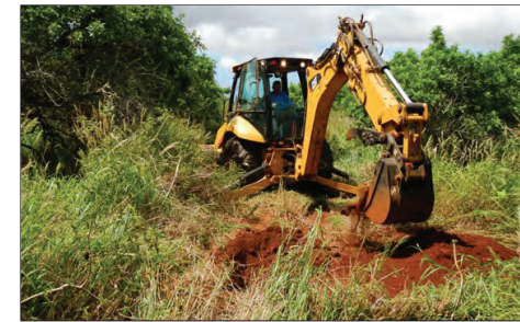
Figure 68: Excavation of Test Pit 15, looking south.
