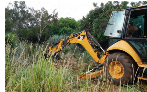
Figure 81: Excavation of Test Pit 23, looking south.
