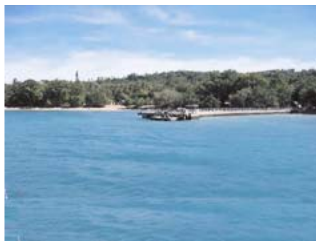
Epi Island—Lamen Bay tender pier
