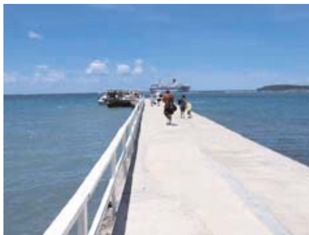
Epi Island—Lamen Bay tender pier
