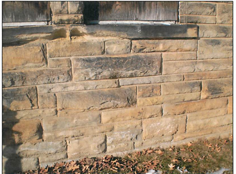
Right side of building (later addition). No diagonally cut stones. 2-24-2015
