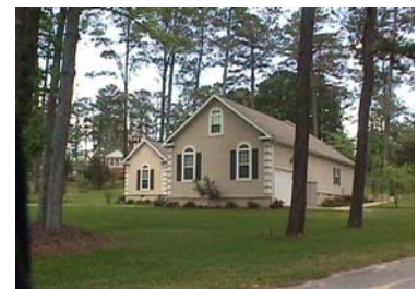
City of Macon Stick Built Residential
