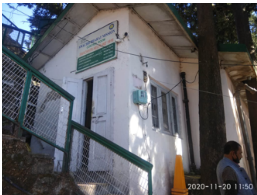
Figure 9: Control room, Shimla City
