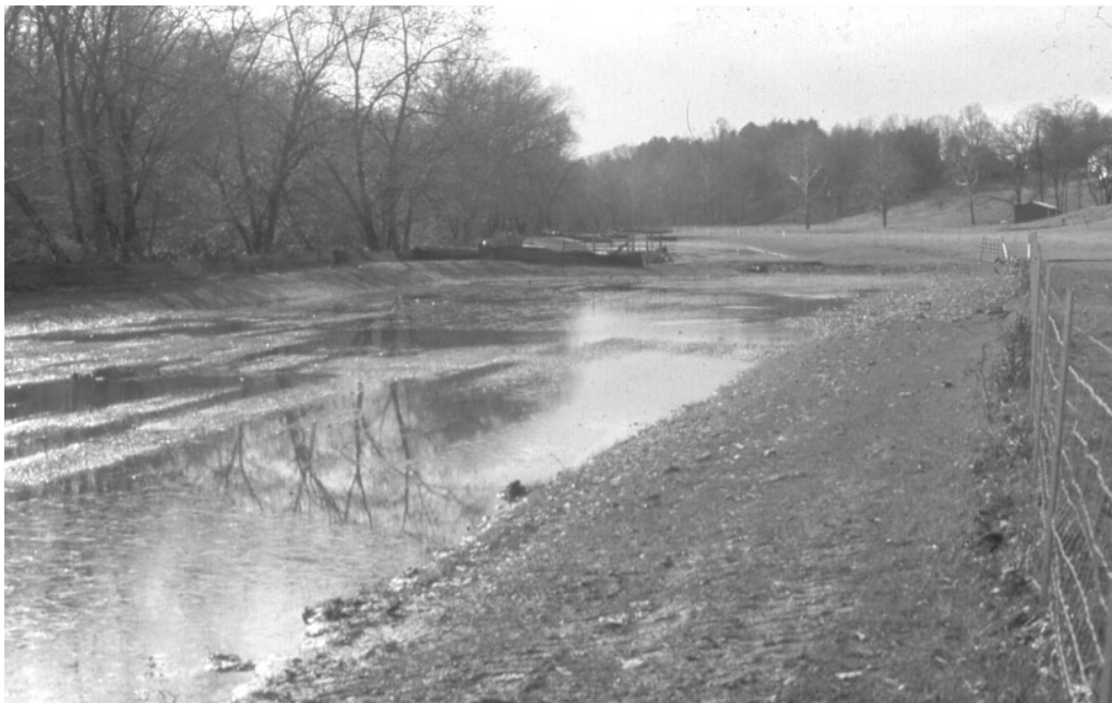
Figure 12-2.—A riparian created wetland made by excavating upland soils down to the presumed winter high water table. This site receives considerable surface and ground water inputs. Excavation of more than 30 in (0.75 m) of soil was required with considerable soil disturbance and compaction. (Photo courtesy of Steve Long, Virginia Department of Transportation. )
