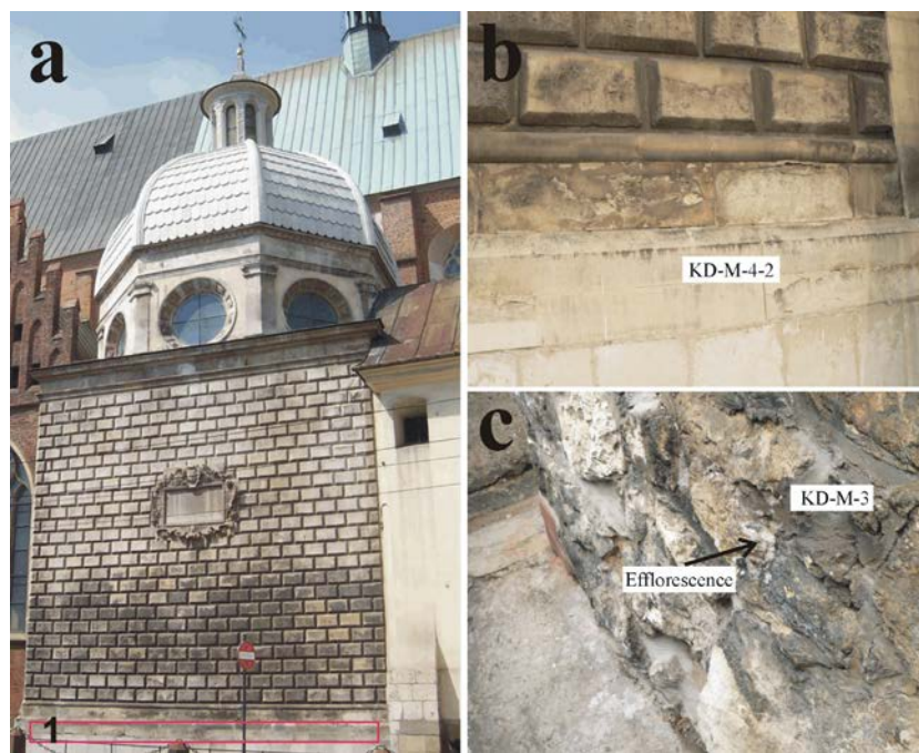
Figure 1. Myszkowski Chapel of the Holy Trinity Church in Cracow (a) and sites of sampling: rusticated wall and elements beneath (b); exposed part of the foundations (c) (after [20], modified). The samples represent: KD-M-4-2—bright, cement rendered part of the elevation; KD-M-3—cement mortar from the subwall, in places covered with salt efflorescence. (1)—sampling area in detail in (b); area presented in (c) is located beneath the pavement level, below the area marked as (1). Photos (b) and (c) by K. Bałaga.
