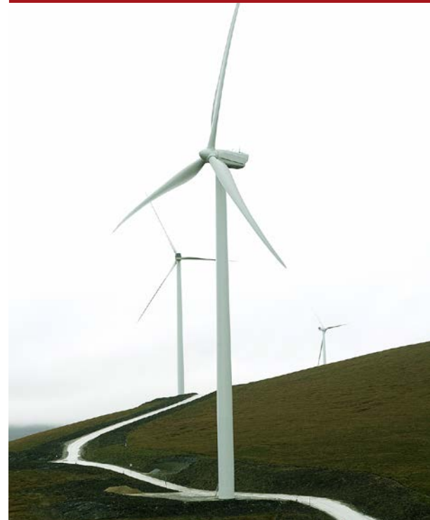
CUTTING THE RIBBON: EDF Renewables has inaugurated its Contract for Difference-backed 177MW Dorenell wind farm near Huntly in Moray, north-east Scotland, featuring 59 Vestas V105-3MW turbines with tip heights of 126 metres
