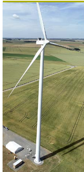
GROWTH SPURT: Epuron commissioned the 17.6MW Torfou wind farm last December
