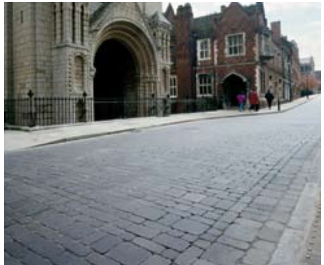
Tumbled blocks combined with a considered range of sizes and muted colours provide an appropriate setting for historic environments such as conservation areas and listed buildings
