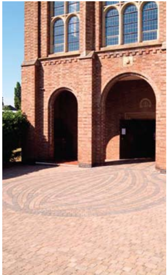
Creation of patterns – whether symbolic, decorative or playful – is natural with precast concrete paving
