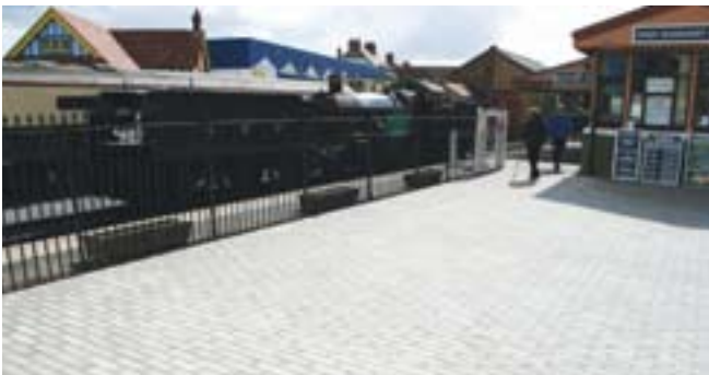
Varied length paving blocks at the West Somerset Railway Minehead Station
