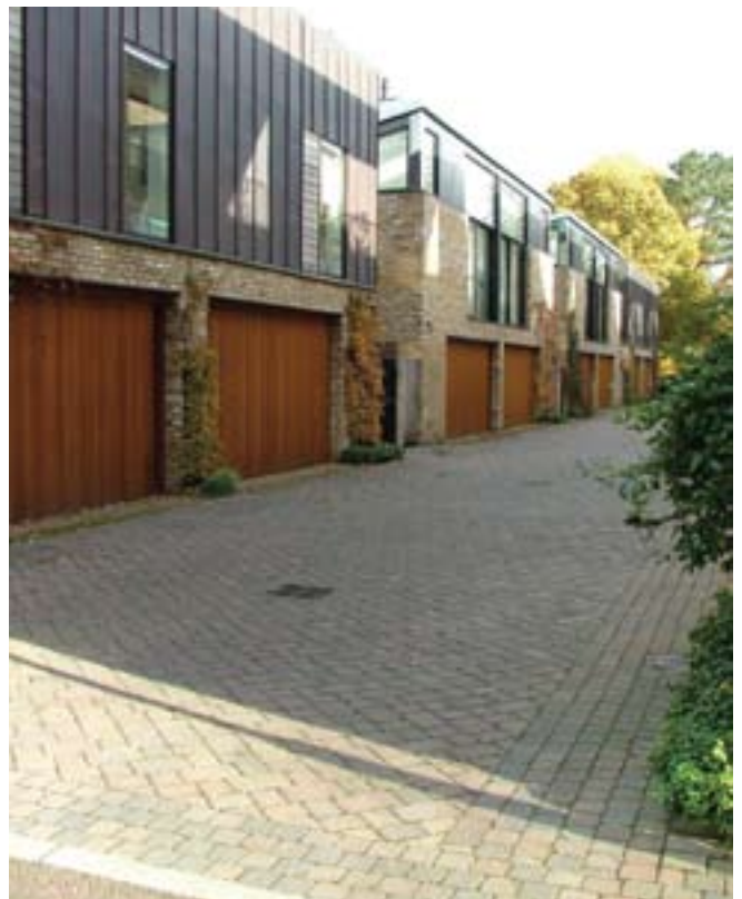
A simple palette of precast concrete paving at the Stirling Prize-winning Accordia housing in Cambridge, made particularly successful by careful detailing and execution
