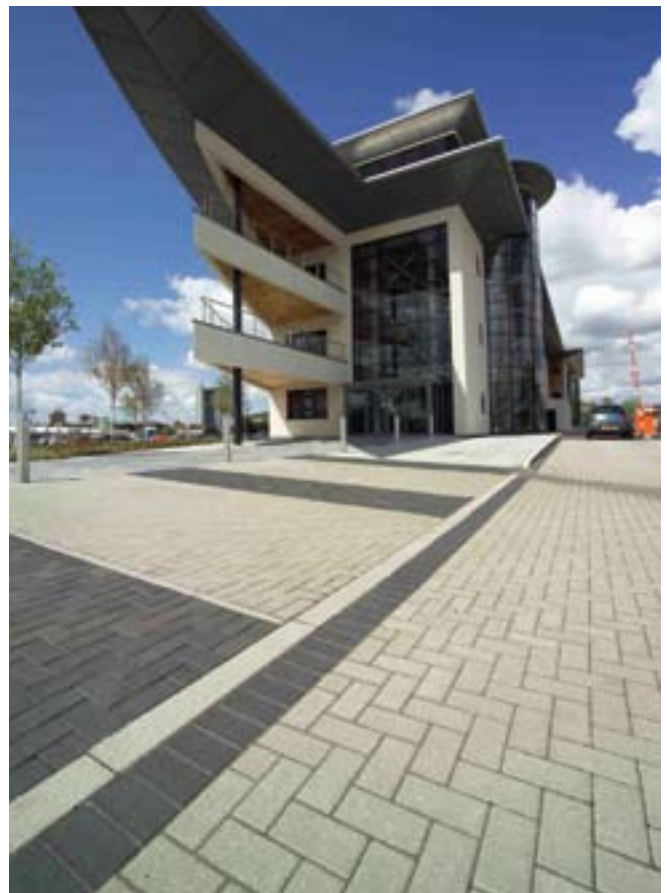
Standard concrete block paving can provide a crisp, regular appearance to suit contemporary buildings
