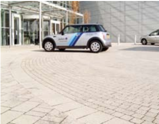
Introducing a contrasting course where patterns change as well as at edges allows a neat transition where cutting is needed
