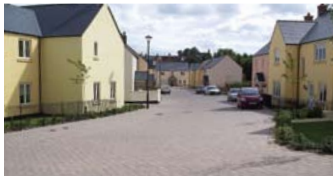
A simple solution to shared surfaces using just one type of precast concrete paving with no delineation of traffic routes, parking or pedestrian areas
