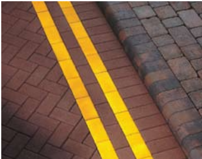
Small element precast concrete kerbs offer additional flexibility with layouts, while factory applied finishes can provide long-term road markings.
