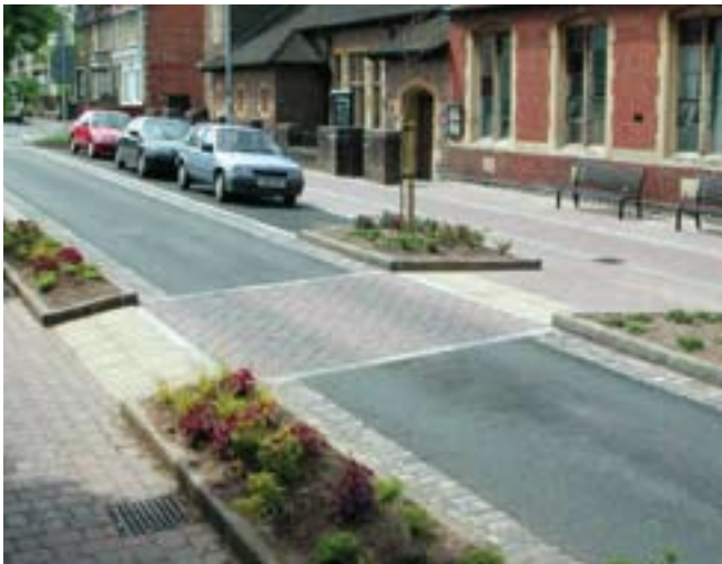
Precast concrete paving provides a change in surface texture and colour to signal pedestrian crossing points, supported by the required tactile paving
