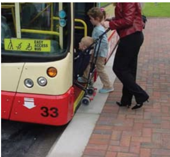
Interpave manufacturers continue to develop innovative products for accessibility for all such as level access kerbs for buses
