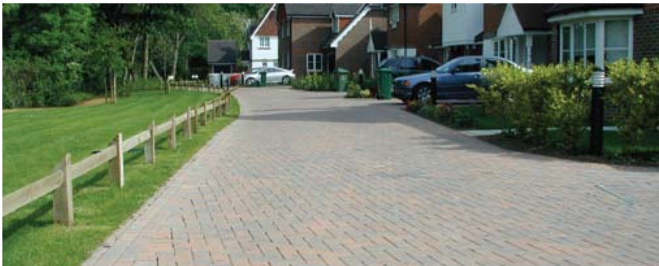
Concrete block permeable paving which has been adopted by a local authority
