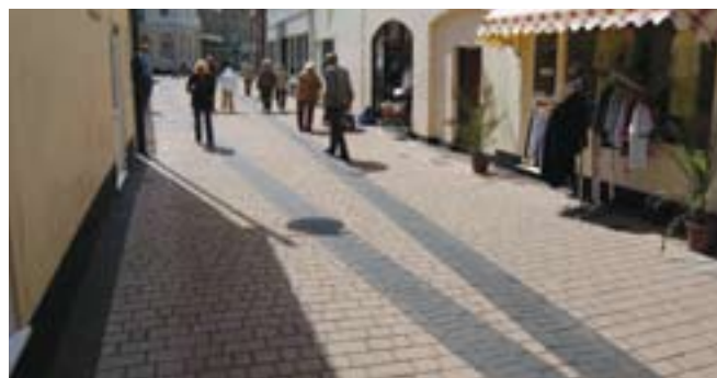
Use of contrasting colour, pattern or texture can delineate routes within shared surfaces while maintaining uniform slip resistance
