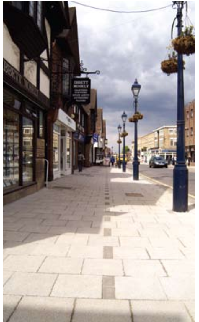
The traditional high street can be simply transformed with wider footways in high quality materials such as these 'granite' precast concrete flags
