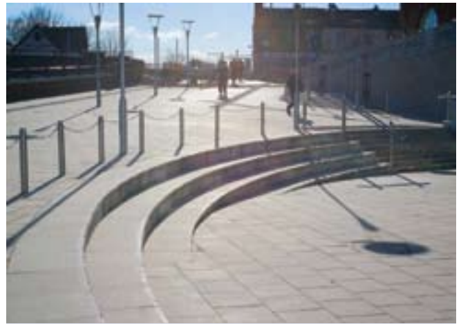
A demonstration of the flexible capabilities of concrete flags to shape external spaces
