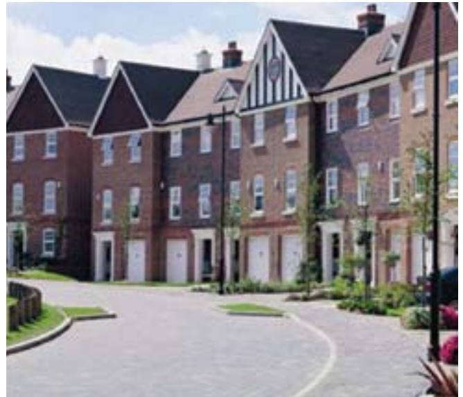
In this housing project, colour and pattern are used to differentiate between highway, footway and crossing points, reinforced by a flush kerb line
