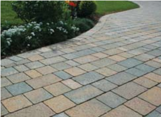
Compared with standard chamfered blocks, concrete block paving today can make use of varying sized modular units with a softer edge
