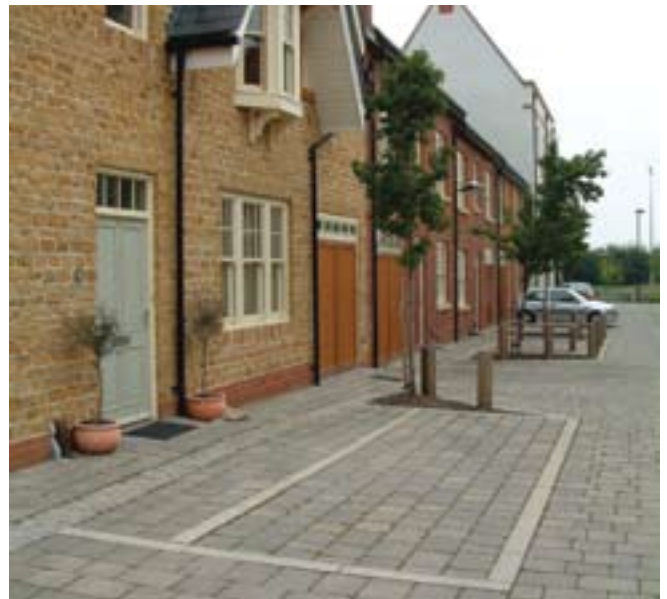
Delineation of car spaces using inset kerb units flush within a single style of block paving at the new Upton development, Northampton
