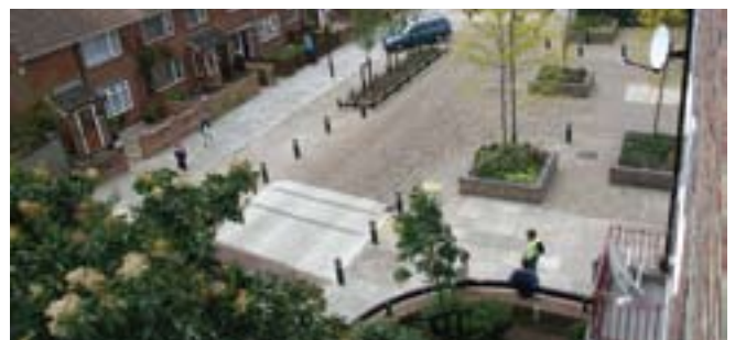
A carefully considered use of precast concrete paving to define distinct areas within a Home Zone in Portsmouth
