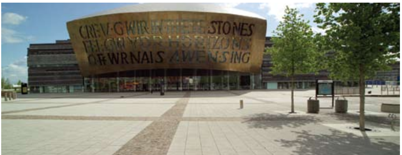
Precast concrete flag paving at the Wales Millennium Centre in the regenerated Cardiff Bay area
