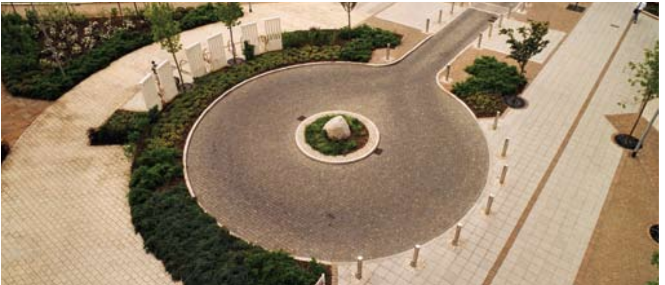
Different styles of precast concrete paving products used in conjunction with planting to create a harmonious design at Teesside University
