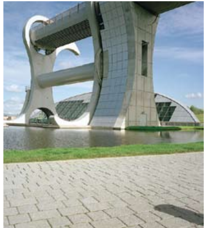
Textured granite aggregate concrete paving at the Falkirk Wheel
