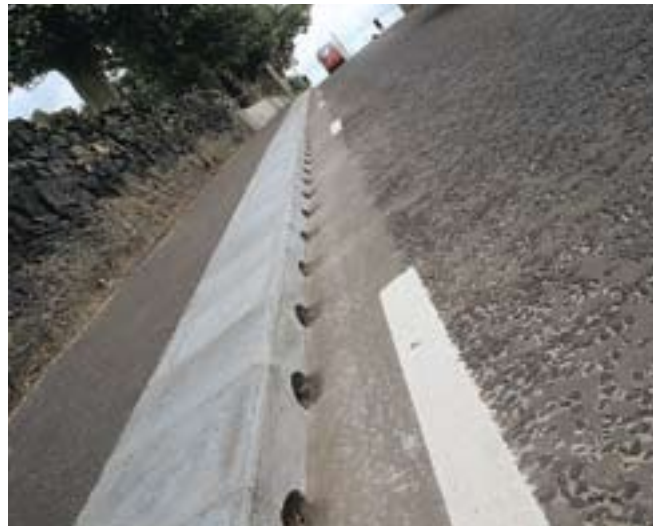
Precast concrete kerbs systems are available with integral drainage facilities
