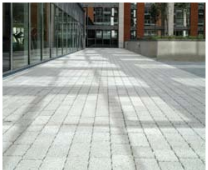
Concrete block permeable paving is also available from Interpave members with enhanced finishes – such as this shot blasted design
