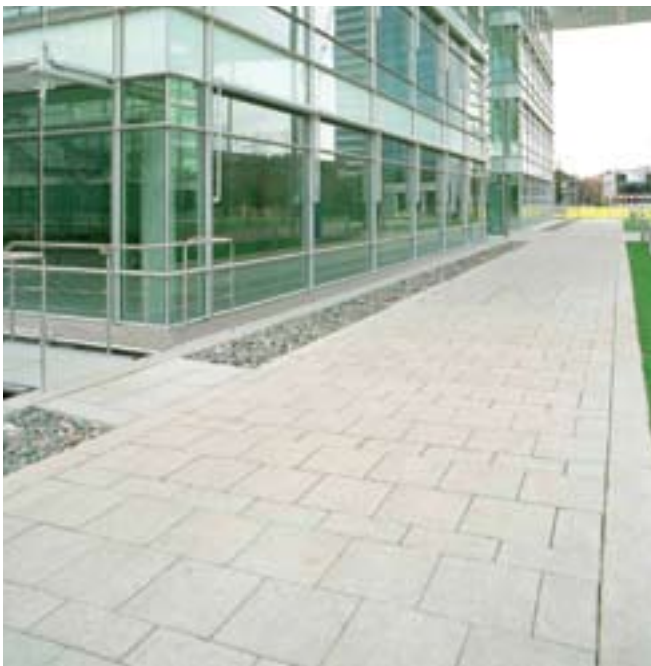
Subtle pattern making using varying sizes of paving and edging units in a single finish while optimising modular dimensions and avoiding cutting
