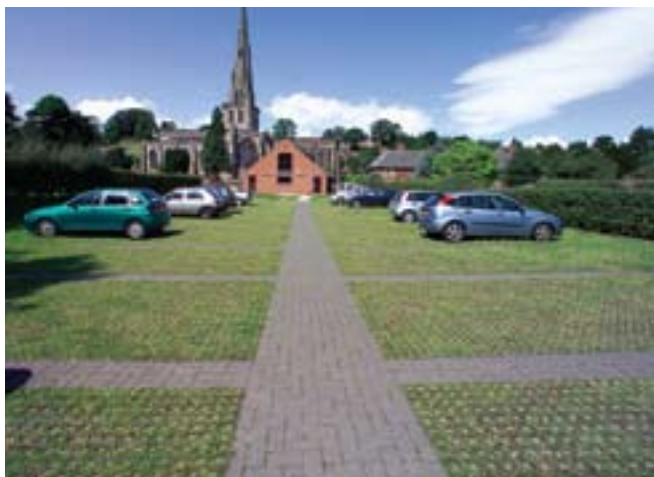
Precast concrete cellular units allow grass growth for a softer landscape appearance while supporting traffic and allowing rainwater to drain through
