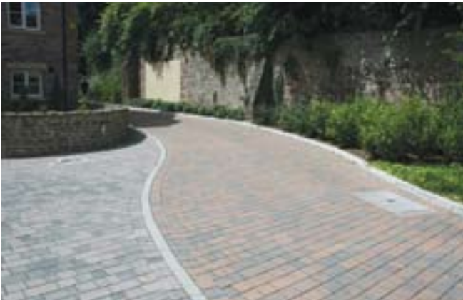
Change of colour reinforced by an inset kerb unit delineates highway from private areas in this shared space
