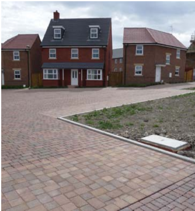
CBPP will be used throughout the 3,300 homes Great Western Park and other major developments in Oxfordshire.
