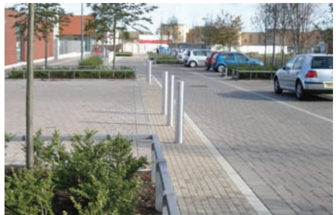
Extensive areas of CBPP used at the Craigmillar redevelopment in Edinburgh – the first to be adopted in Scotland. A case study on this project can be downloaded from www.paving.org.uk
