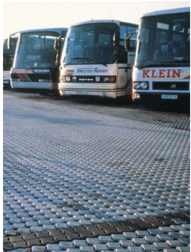
Extensive areas of concrete block permeable paving for bus parking areas installed in 2000 at the World Exposition, Hanover.
