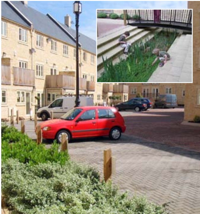
CBPP at this housing scheme in Stamford supplies clean water to landscape features.
