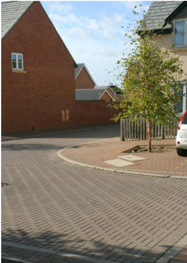
Monitoring of the Cambourne project highlights the robust performance and minimal maintenance needs of CBPP.
